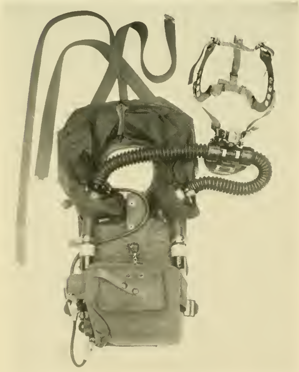
Fig 14.10 The Westinghouse Min-O'Lung (left) and Drager (right) emergency breathing systems. Both have about 0.5 hours endurance. (Westinghouse Corp.)
